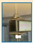
Standard method using nuts and washers.
