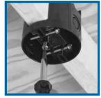
Just one hand is required to mount the box using the pre-located mounting screw.
