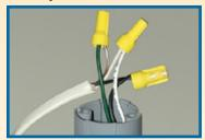
Connect receptacle wires to romex. Be sure to match wire color(s).
