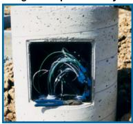
Once your J-Boxes are installed, you can speed projects along by pre-wiring before poles arrive. Or, you can install poles first and use them to mount cable-pulling equipment — a particular advantage for long, difficult wire pulls. Of course, all the extra hand room our J-Boxes offer makes splicing much easier and faster than working through cramped pole-access holes.
