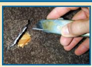
Cut 2%" hole through carpeting before using hole saw.
