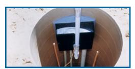
J-Box, with all conduit and fittings placed as desired, is temporarily attached to the concrete form - base
