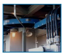
Horizontal (suspended) tray, with vertical drop to machinery below
