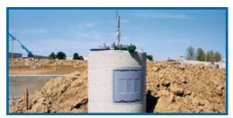
Remove form after concrete has been poured and allowed to cure.
